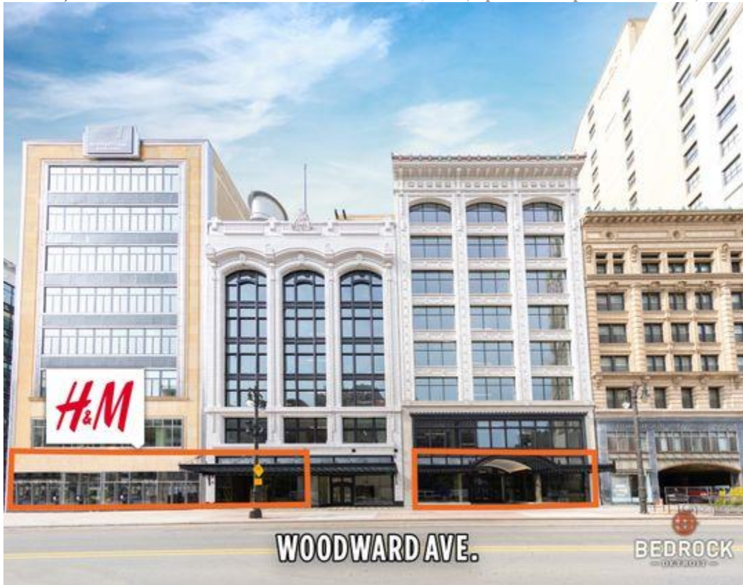
Finished exterior facade of 1515 and 1529 Woodward before retail tenants move in on September 27th, 2019 (Photo: Bedrock Detroit)
